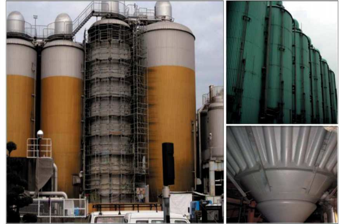
Atometal AM-C Result of Kirin Beer Tank Coating
